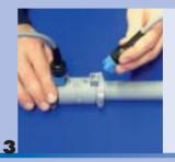
Fit the cable plugs of the welding tool onto the sleeves provided.
