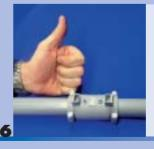
Remove cable plugs; the connection is now fully welded.
