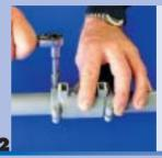
Join pipe and fitting, and tighten the screws.
