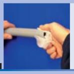
Thoroughly clean the outside of the pipe ends and the inside of the connection elements using BEKOFLOW® cleaning cloths.
